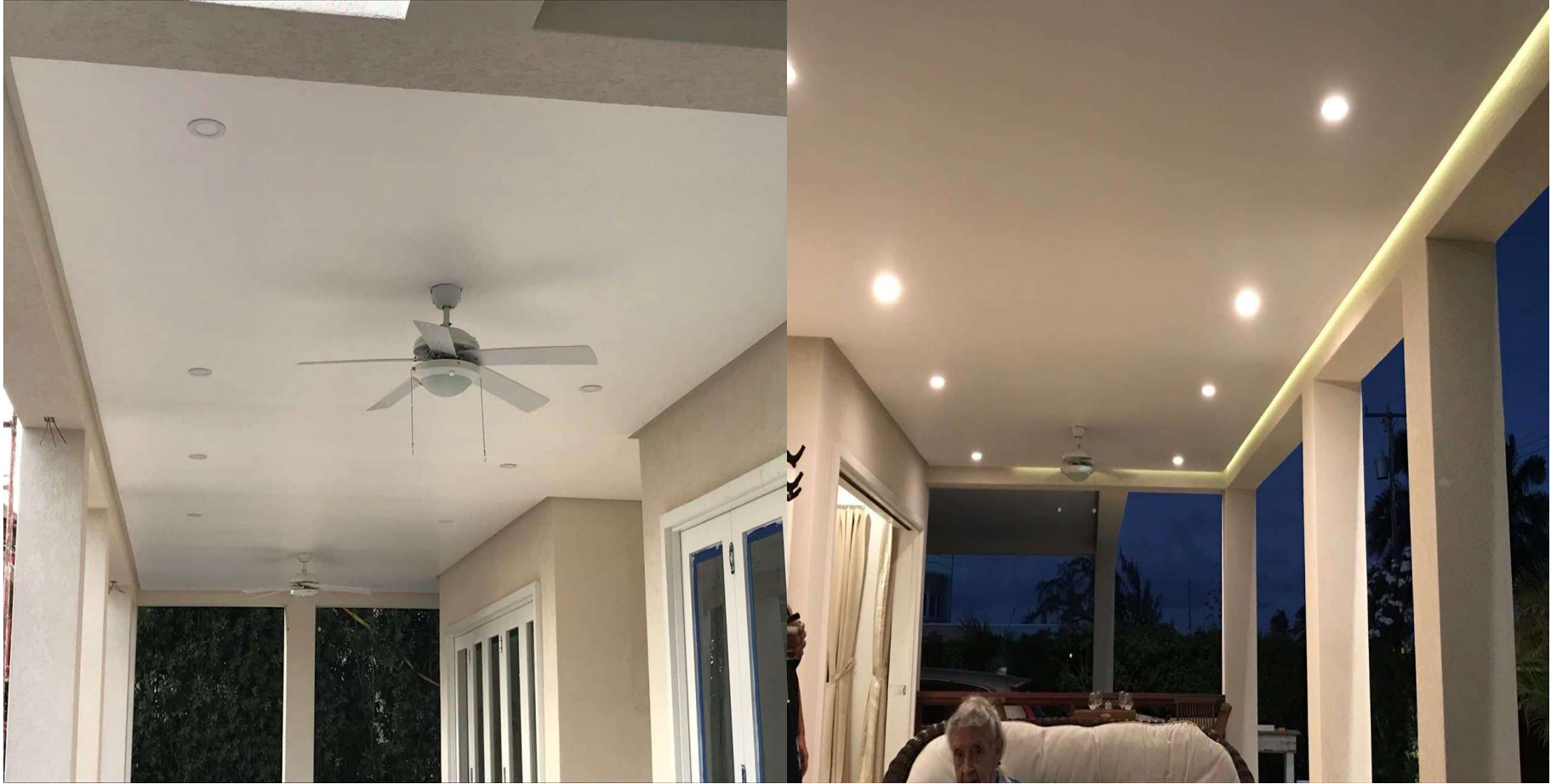
Sigma Plaster Trim 50 x 50mm with concealed LED strip - Atlantic Shores
